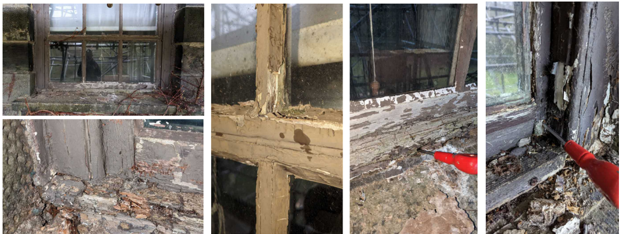
Images showing extent of timber decay at cills, glazing bar joints and jambs
